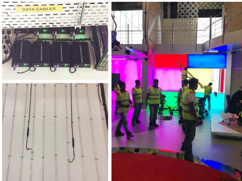
Photos of the studio's colour-changing panels – backlit with RoscoLED Tape VariColor
