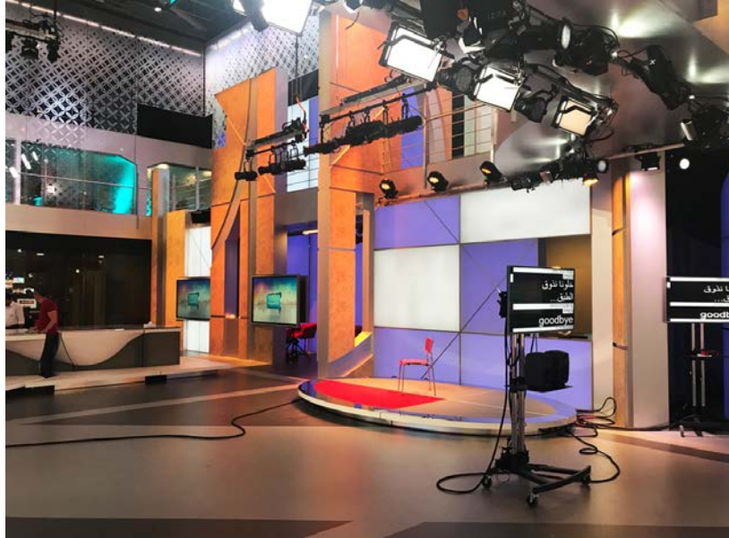
Rosco Silk 210 LED Soft Lights provide even illumination, while RoscoLED Tape VariColor backlights the wall panels in lavender & white
