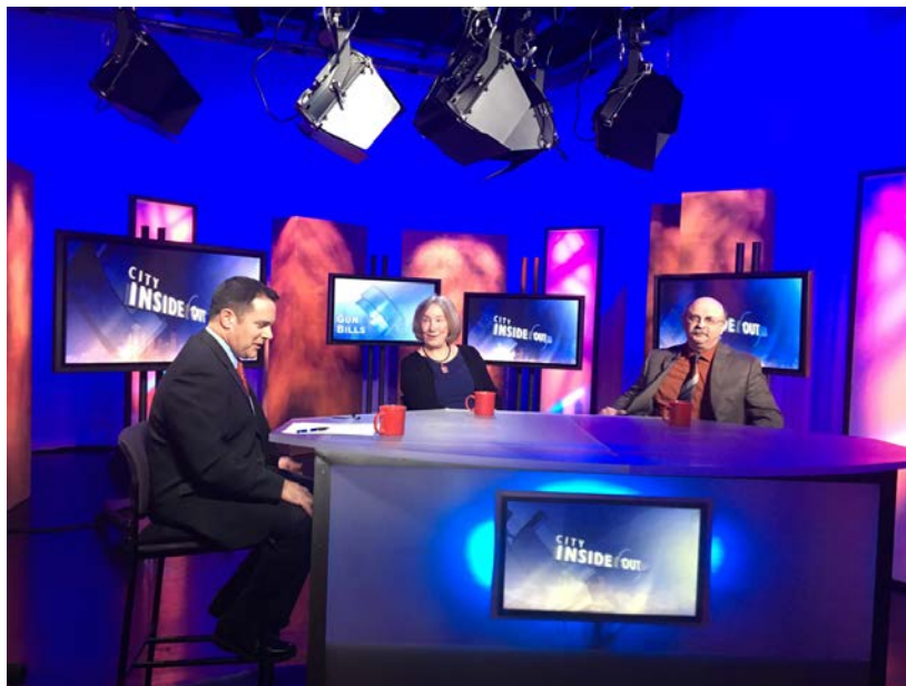
The results of Seattle Channel's LED lighting upgrade
